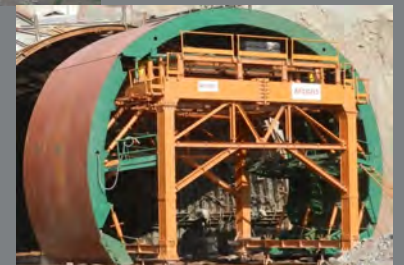
Figure 2: Gantry for Concrete lining of Wider Section Tunnel
