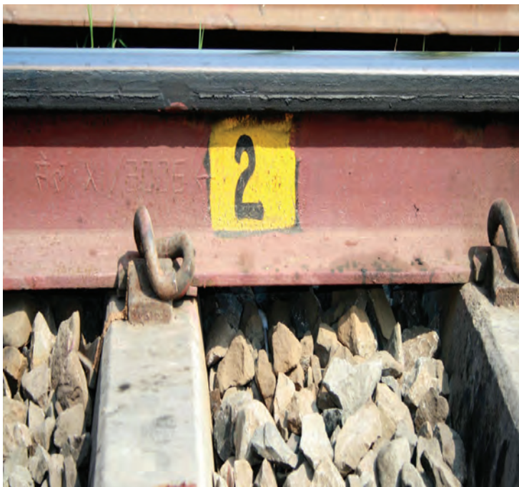
Fig. 2.9 : Lubricated outer rail of curve
