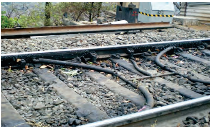
Fig. 2.10 : Automatic curve lubrication
