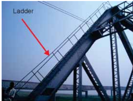
Fig 1.6: Ladder is added to end frame to reach up of through only
