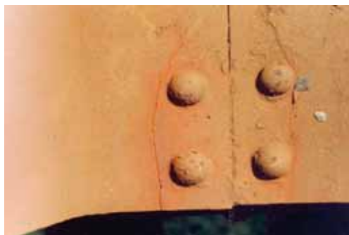
Fig. 2.38 Development of crack at riveted connection
