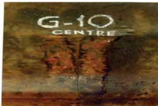
Fig. 2.37 Crack and Corrosion at sleeper seat
