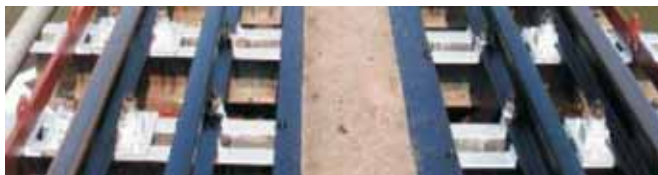
Fig. 2.45 Fixing of guard rail
