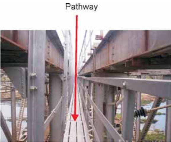
Fig 1.5: Pathway for inspection from side of the bridge
