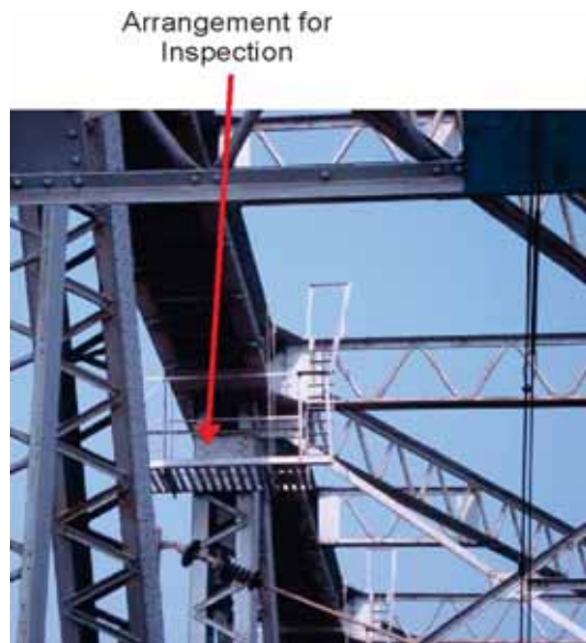
Fig 1.7: Arrangement for inspection on top chord
