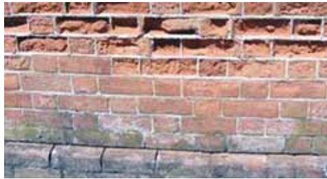
Fig. 2.8 Weathering of masonry block
