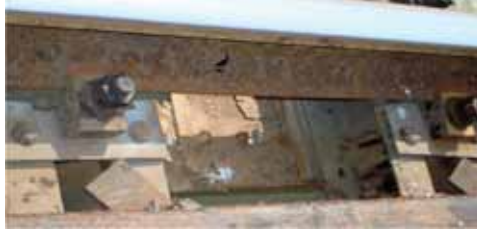
Fig. 2.34 Corrosion of top flange due at seat sleeper
