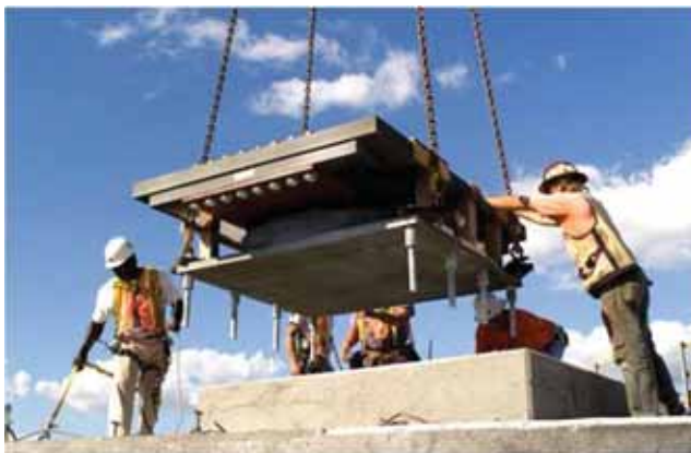
Fig. 2.31 (b) Installation of Pot-cum PTFE bearing
