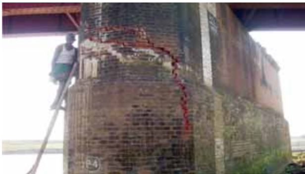
Fig. 2.5 Cracks in masonry piers
