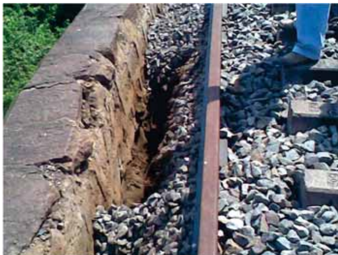
Fig. 2.18 Bulging and/or tilting of the spandrel walls
