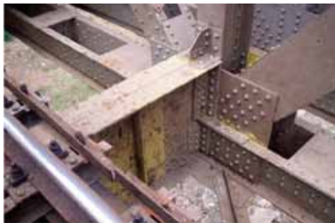
Fig. 2.35 (b) Corrosion at riveted connection
