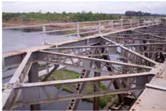
Fig. 2.36 Rivet connections of bracing with top boom
