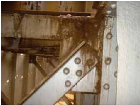
Fig. 2.35 (a) Corrosion at riveted connection
