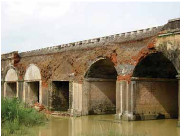
Fig. 2.20 Collapse of face wall
