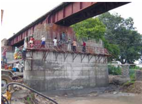
Fig. 7.7 Jacketing of bridge pier in progress
