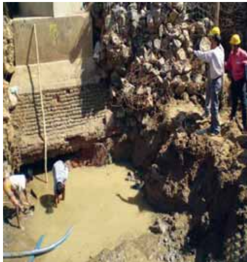
Fig. 2.3 Effect of scour on a shallow foundation
