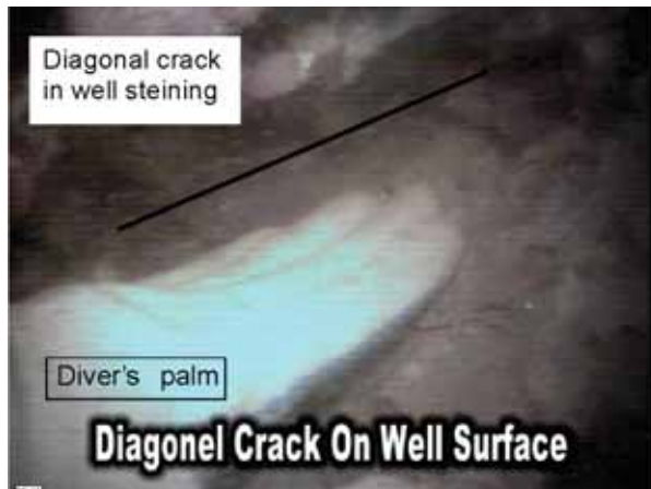
Fig. 3.3 Digonal crack in well steining
